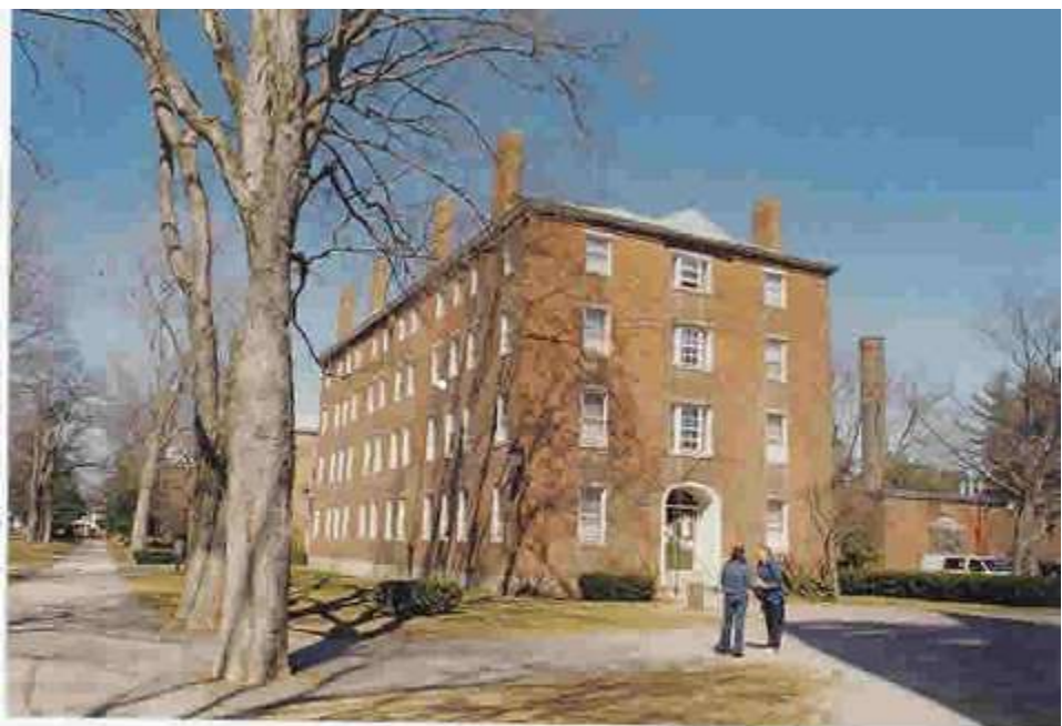
Maine Hall, Bowdoin College, Brunswick. Built in 1808 and originally known as the College. Rebuilt in 1836.
