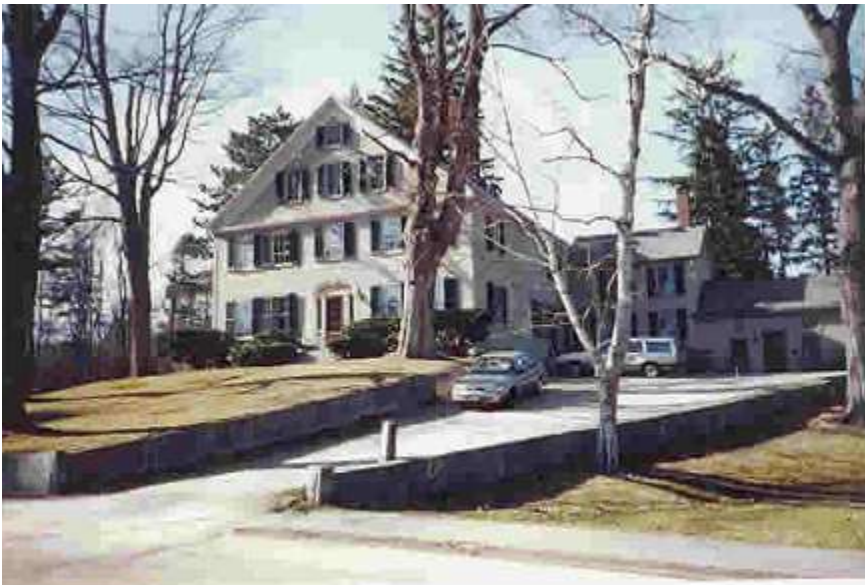
Walker - Wilson House, 2 Melcher Place, Topsham. Built in 1802 - 1803. Legend has it that this was a safe house.
