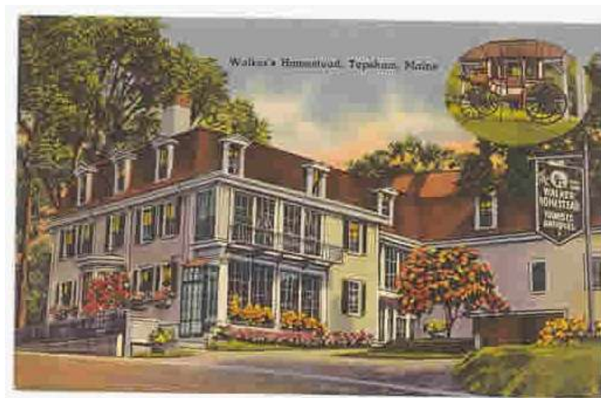
Walker Homestead, 1 Elm Street, Topsham. Built in 1808 - 1809 and used as an Inn. Tunnels lead from the cellar to the Charles Thompson House and the General Samuel Veazie House. Torn down in the 1960's
