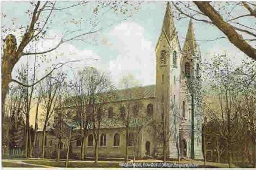
Kings Chapel, Bowdoin College, Brunswick. Built 1845 - 1855. The Chapel is also known as Bannister Hall.
